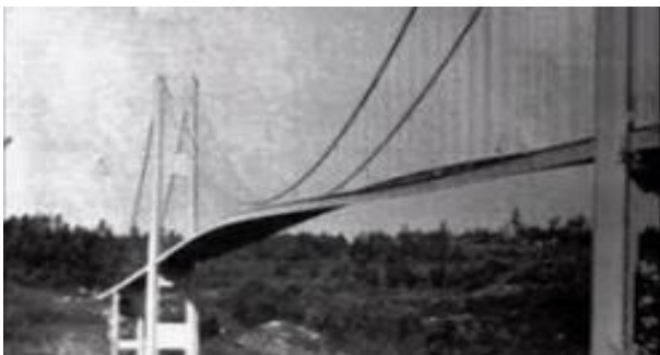
[Fig.2: Old Tacoma Suspension Bridge] [18]
